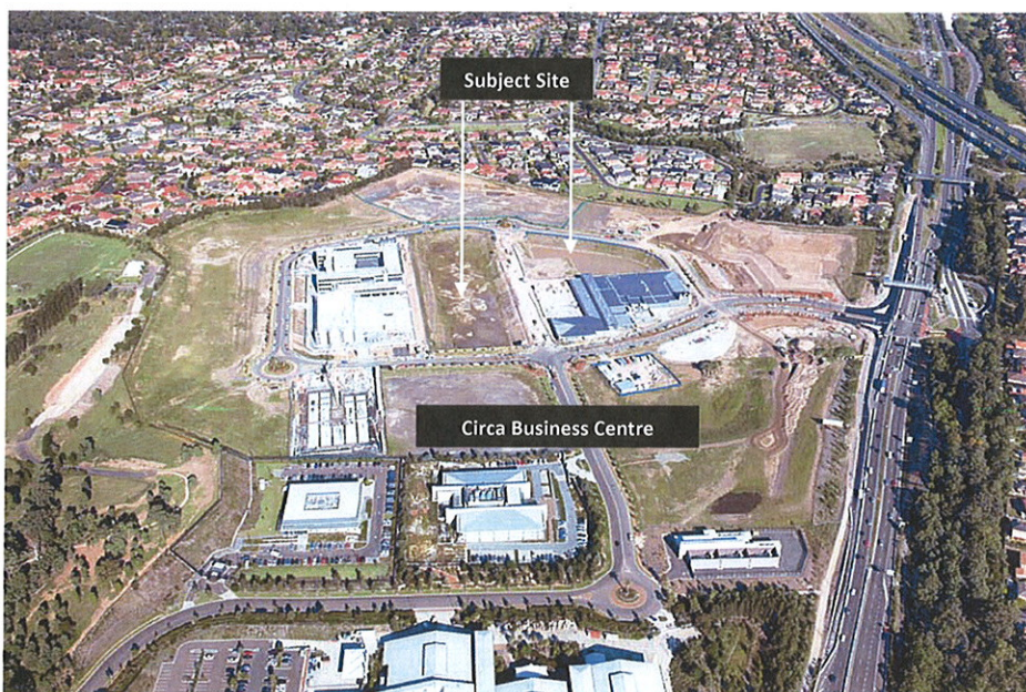
Aerial Photograph of Site - April 2009
